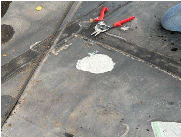
Core sample sealed up
