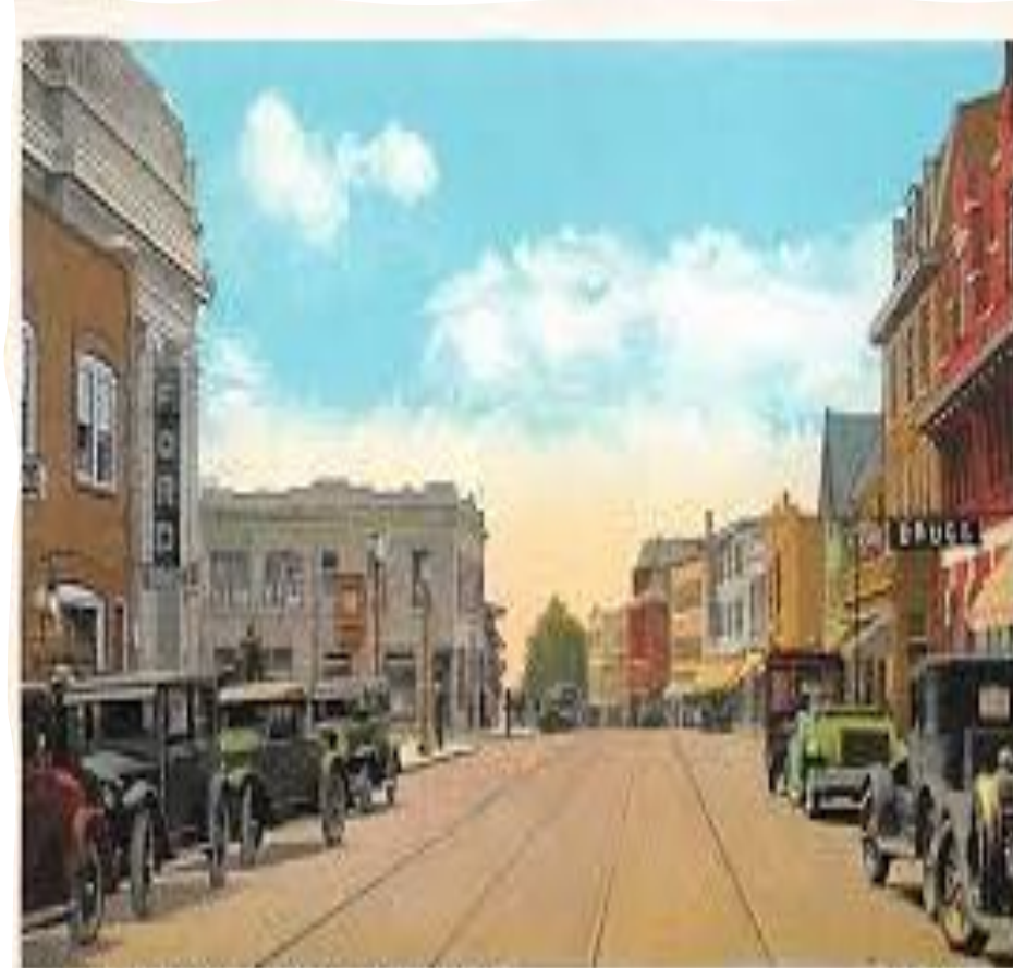
14 YORK ROAD, LOOKING SOUTH, JENKINTOWN, PA
