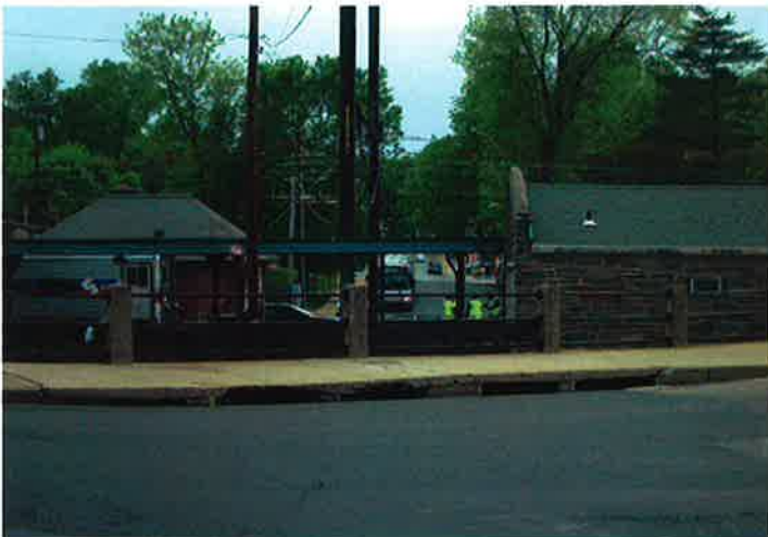
Multiple storm drains are required at the train station
