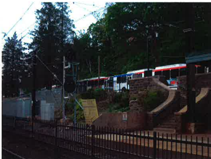
Jenkintown-Wyncote Train Station
