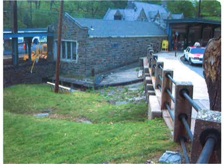
Drainage down this hill requires multiple drains, and the site has flooded in the past
