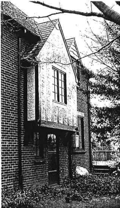
Wood brackets, mortice and Tenon joints in timbers.
