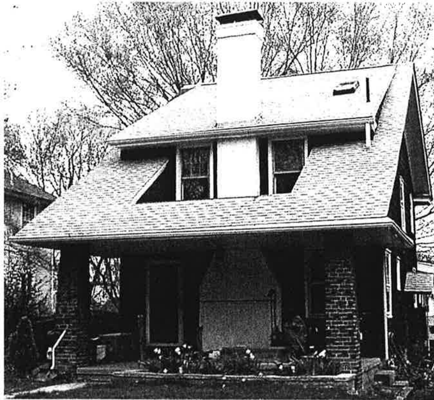
Craftsman bungalow with battered brick columns. Note the irregular work in the columns.
