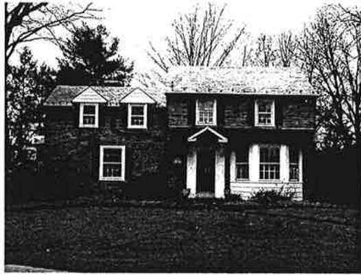
Colonial Revival in a Mid Atlantic English form. Note the pent roof over the bay window.
