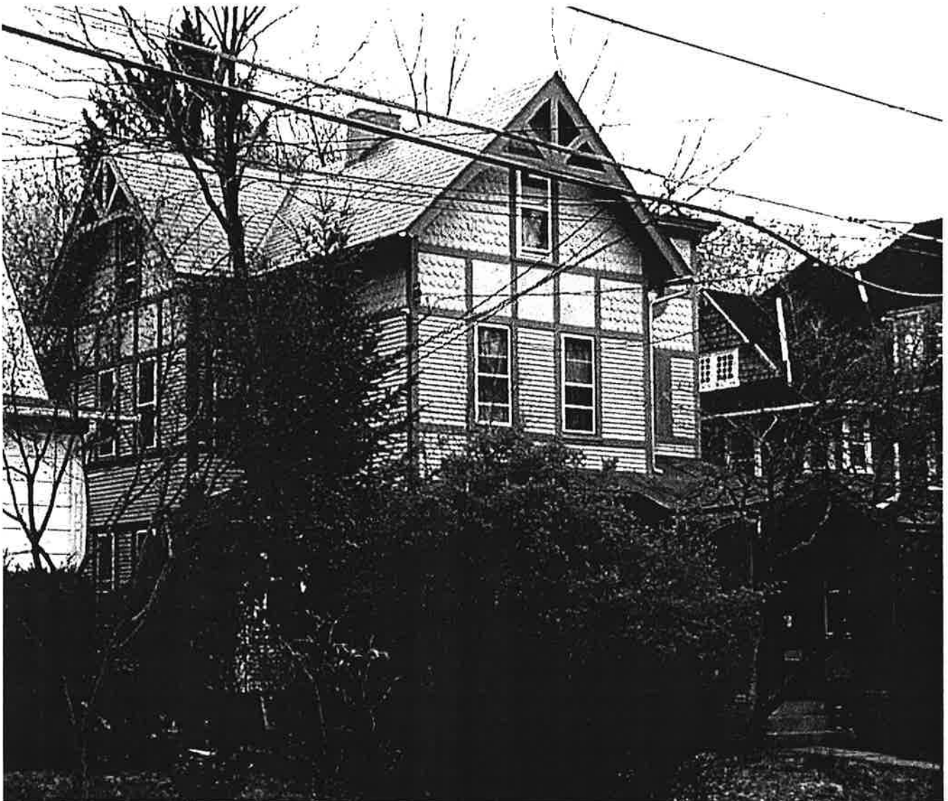
Eastern Stick style with cross gable roof and tower. Note the simulated structure with a variety of shingles and siding.
