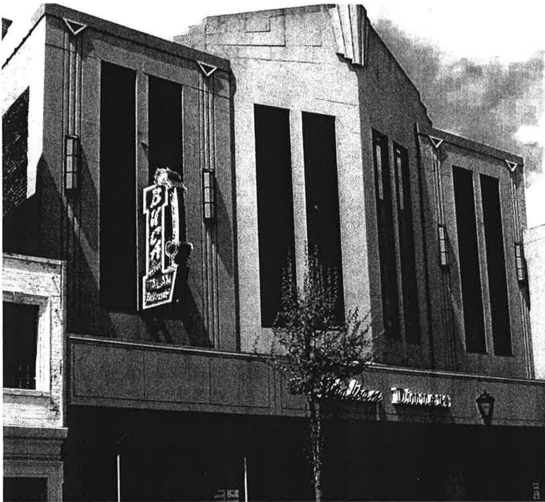
Art Deco commercial structure with window registers and vertical fluting.
