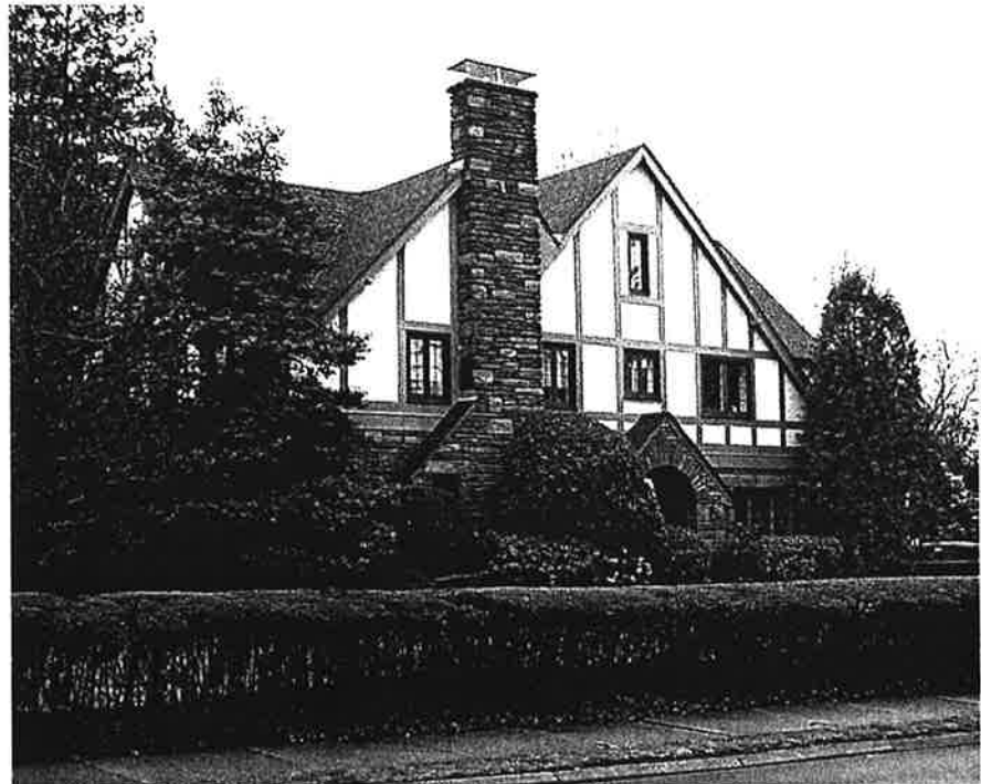
Stucco Infill with faux half timbering.
