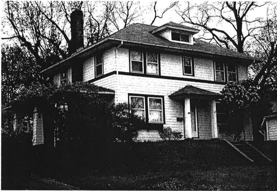
Craftsman Four Square with shirtwaist belt-rail and battered shingled columns on side porch.
