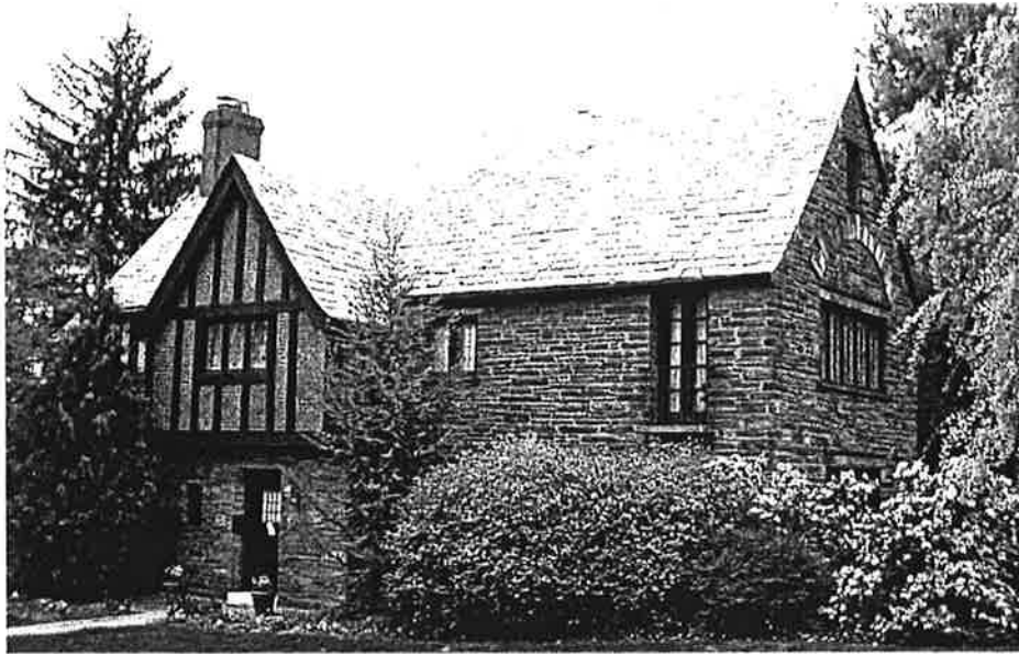
Stone Tudor with projecting 2 nd floor bay featuring half timbering and brick nogging.
