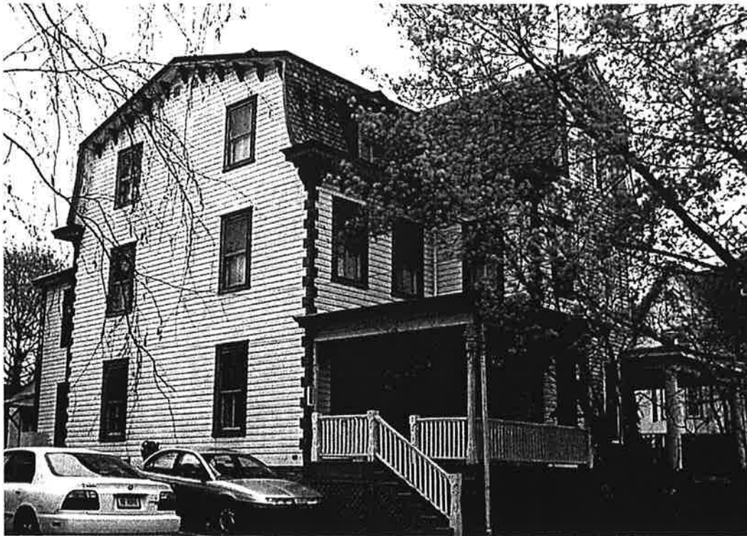
Second Empire twin with painted wood quoins at corners and gambrel roof simulating a mansard Roof.
